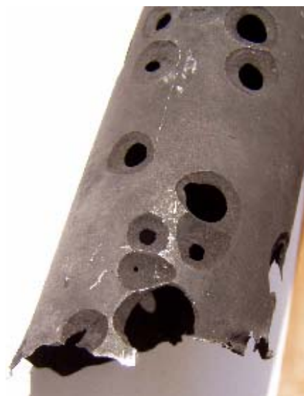
Fig. 2. A general view on the inlet tube made of Alloy 800.
